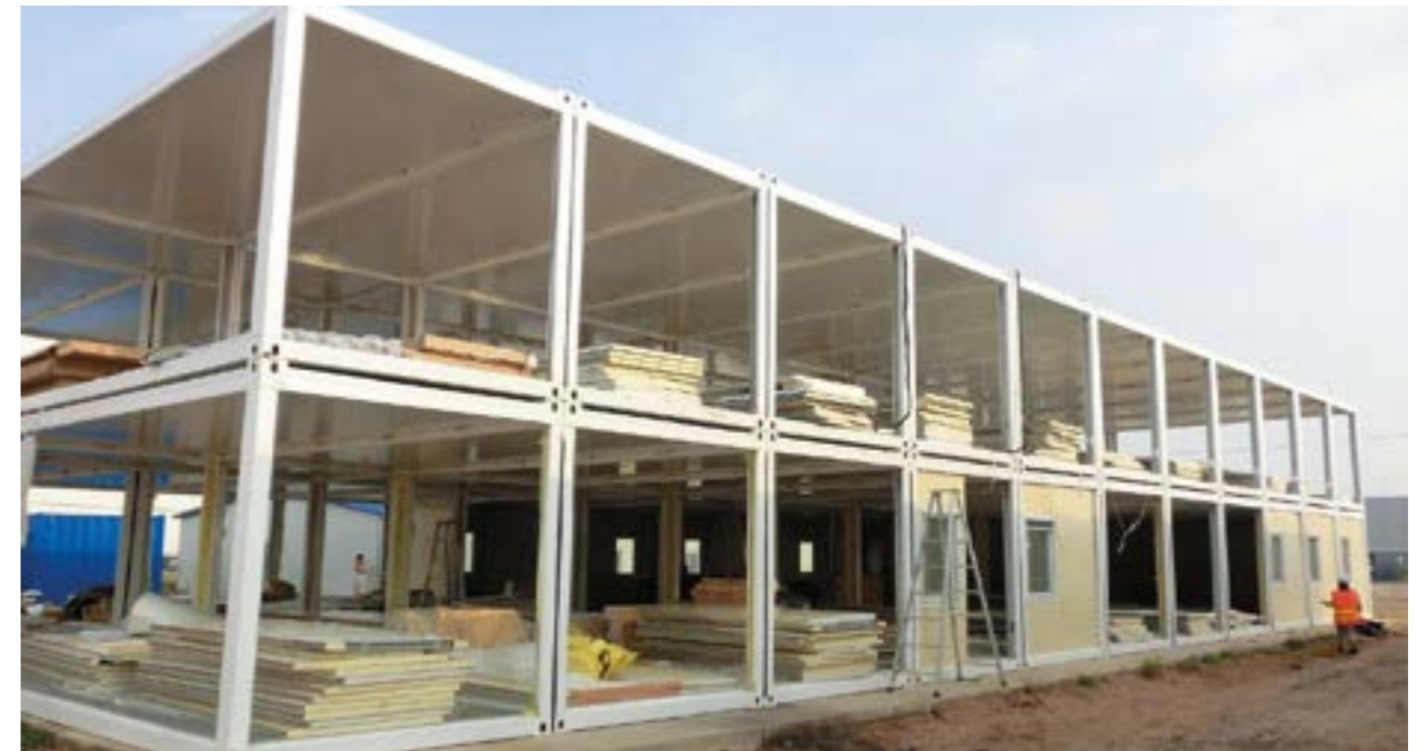
Example of modular construction for emergency situations
