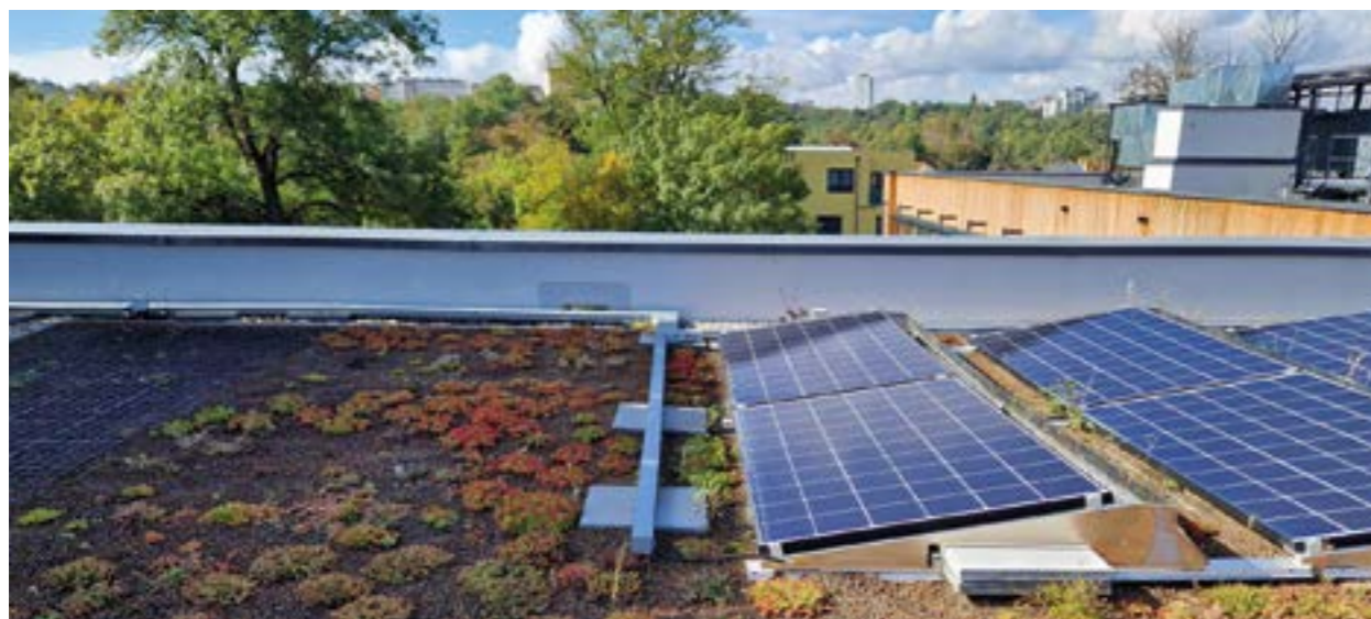
Example of a bio-solar roof, school building in Prague 9, © Ecoten
